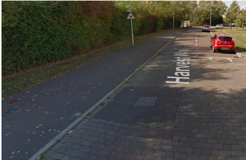
Figure A. 14 – Existing facilities “6” (looking northwest along Harvest Way)
