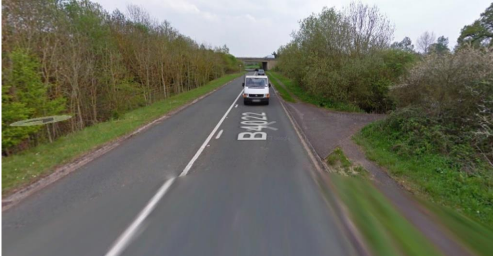
Figure A. 24 – Proposed facilities “13” (looking southeast along the B4022 at the shared use narrow path on the south side)
