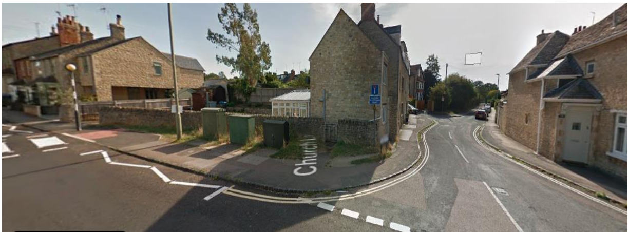
Figure A. 25 – Proposed Improvement 14 (looking south at the entrance to Church Lane). Potential to drop kerbs at mouth of junction to Oxford Hill (B4022).
