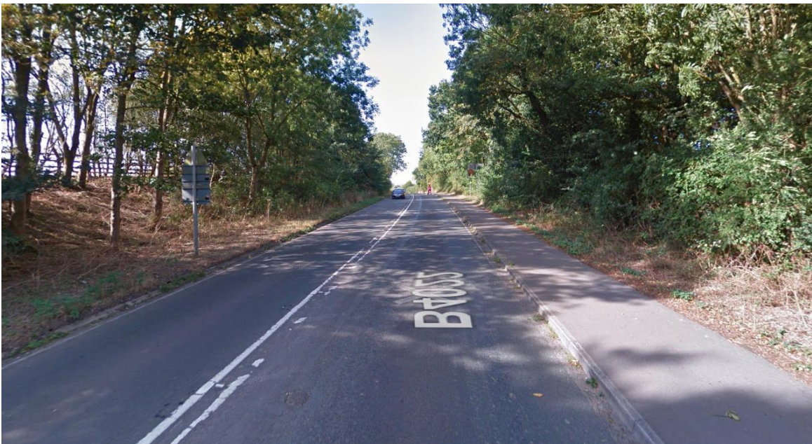
Figure A. 23 – Proposed facilities “12” (looking northwest on Oxford Hill at the shared use cycleway on the north side)
