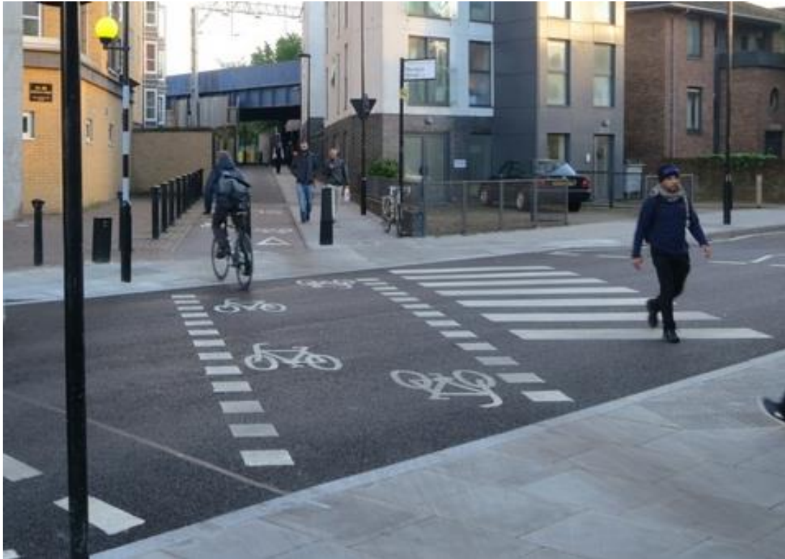
Figure 12 – Example of a Parallel Crossing in London (also referred to as a “Tiger Crossing”).
