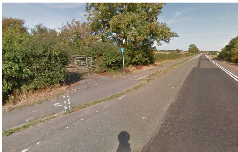
Figure A. 16 – Existing facilities “8” (looking northeast along the A40 slip road at the shared use cycleway)
