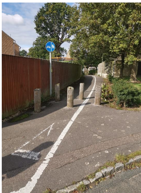
Figure A. 7- Barriers at Blakes Avenue crossing on RoW route 410/41
